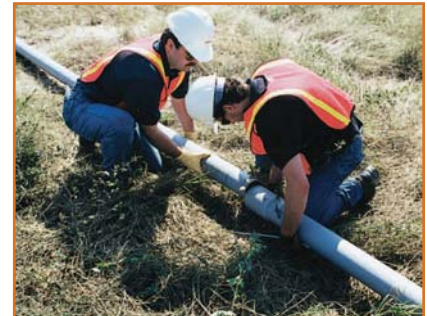
Attach the next piece of Bore-Gard.
