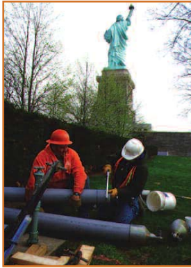
Trim spigot end before attaching pulling eye.
