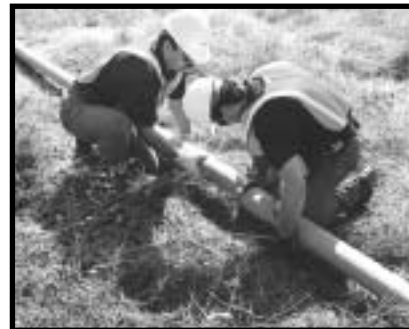
Attach the next piece of Bore-Gard.
