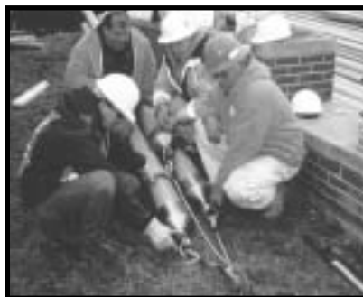
Tighten pulling eye so that it expands against interior of the conduit.
