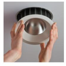
**Step 5:**Gently press upward until the downlight is snug against the ceiling.
