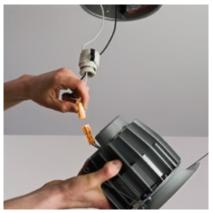
Remove one of the screws from the existing housing and place the ring terminal from the green bonding wire under the screw and retighten the screw to the housing. Plug the male end of the socket adapter into the female end that is attached to the downlight.
