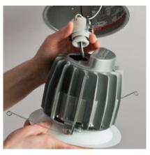
Step 3: Secure the socket assembly to the top of the downlight by pressing the sides of the black springs and inserting them into the notches on the top of the bracket.
