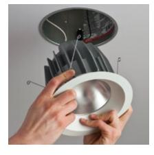
**Step 4:**Compress the springs on the side of the downlight and insert them into the brackets on the inside of the pre-installed recessed housing.
