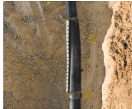
4 Finished sleeve is moisture resistant and durable.
