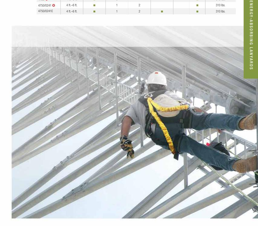
The SafeAbsorb lanyards include 6 foot web and cable offerings with external energy absorbers that meet ANSI Z359.13-2009 standards. Available with snap hooks and/or rebar hooks, allowing for a variety of attachment options. 3,600 lbs. gate rated hardware.
